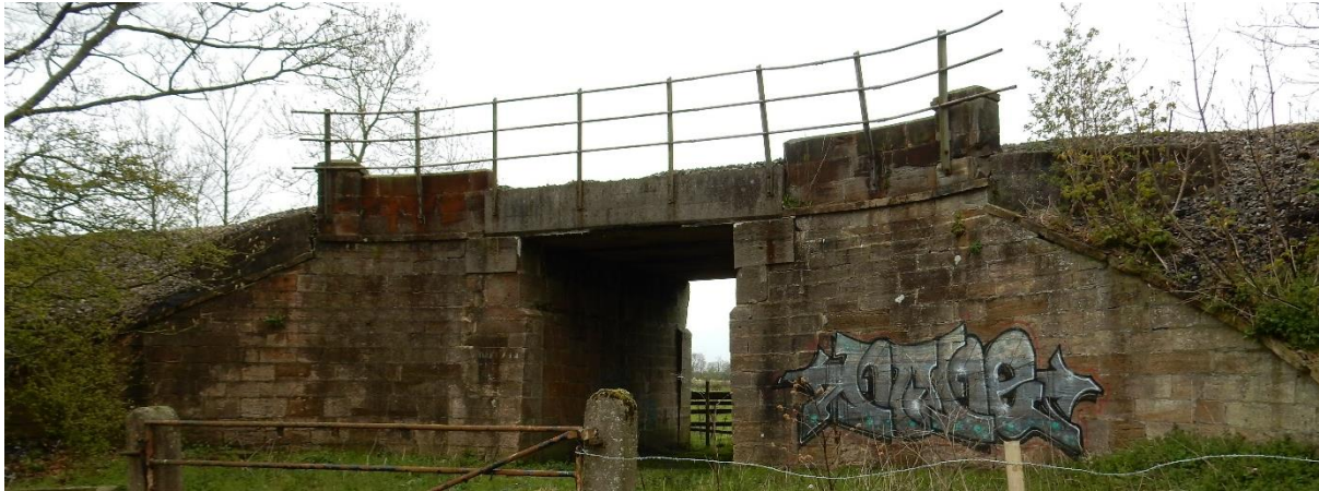
Plate 22. Myers Flatt Accommodation Bridge with its replacement decking, probably added 1901.
