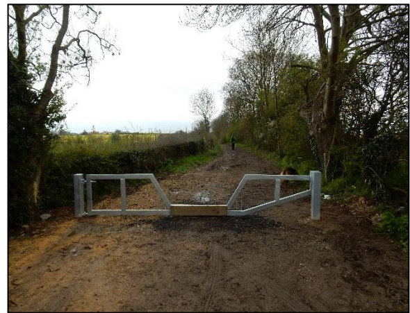
Plate 31. Left: New cycle paths south of Newton Aycliffe are being used for fly tipping. Right: barriers at entrance points to bridleways ensure that pedestrians and horses can access the path but vehicles cannot. However, it also excludes mobility scooters.
