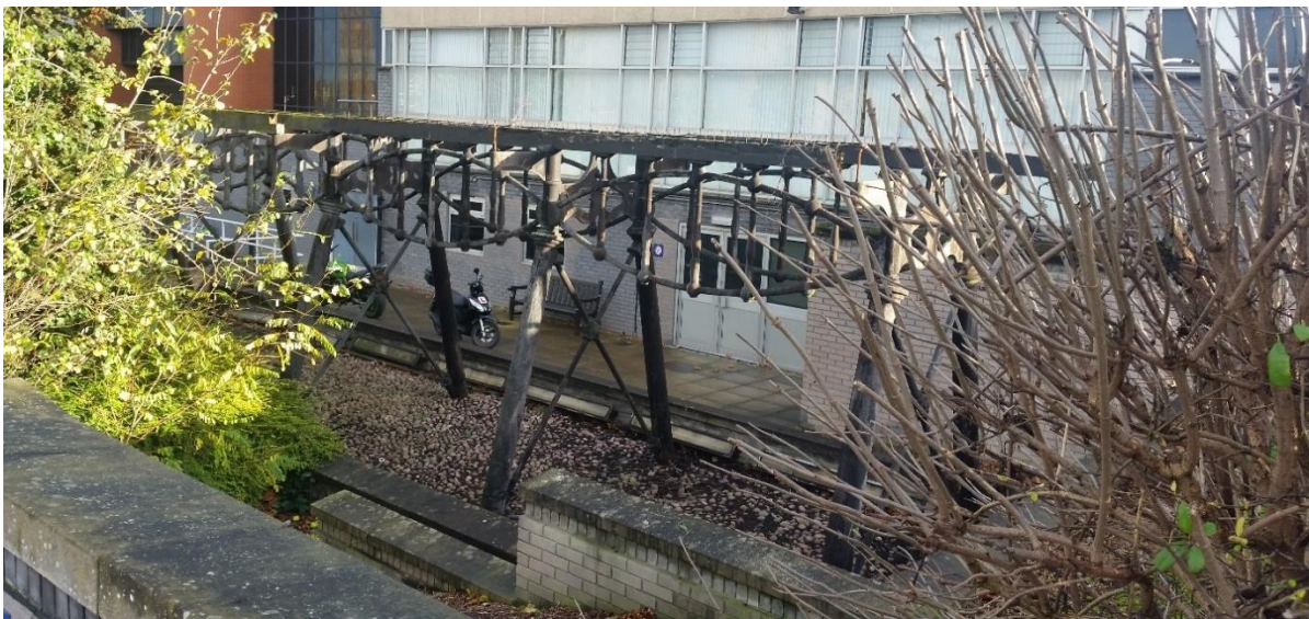
Plate 20. The ironwork at the National Railway Museum in York – this should be moved to the National Railway Museum in Shildon
