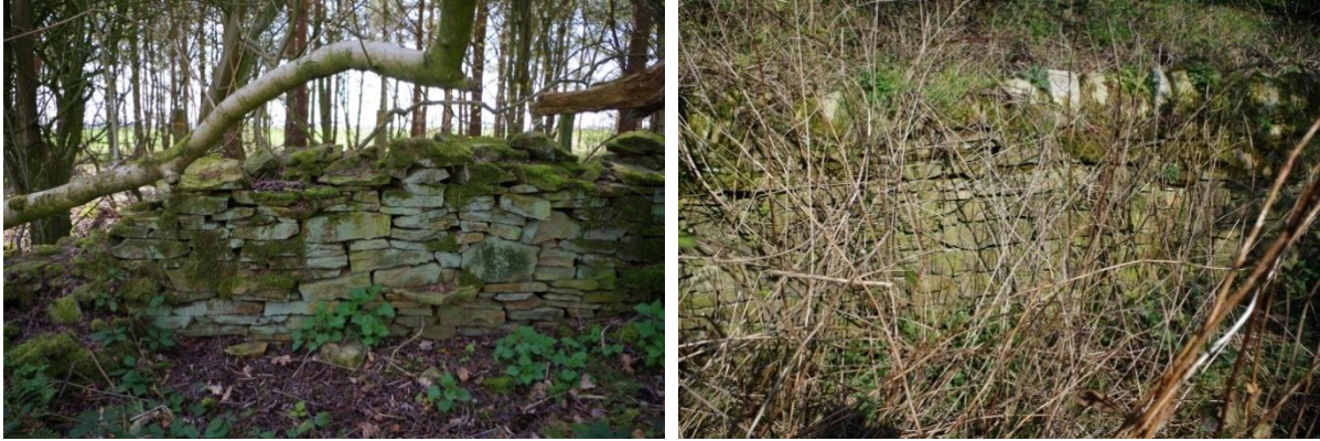
Plate 10. Examples of surviving S&DR boundary walls. The one on the right was behind barbed wire but survives to full height with triangular coping stones.
