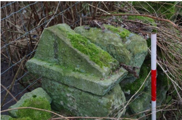
Plate 9. (above left) A two-hole stone sleeper from Etherley Incline and (above right) another incorporated into a dry stone wall near the site of the Engine House. Several architectural fragments from the now demolished engine house and cottages are present on site and re-used in boundary walls (below left).
