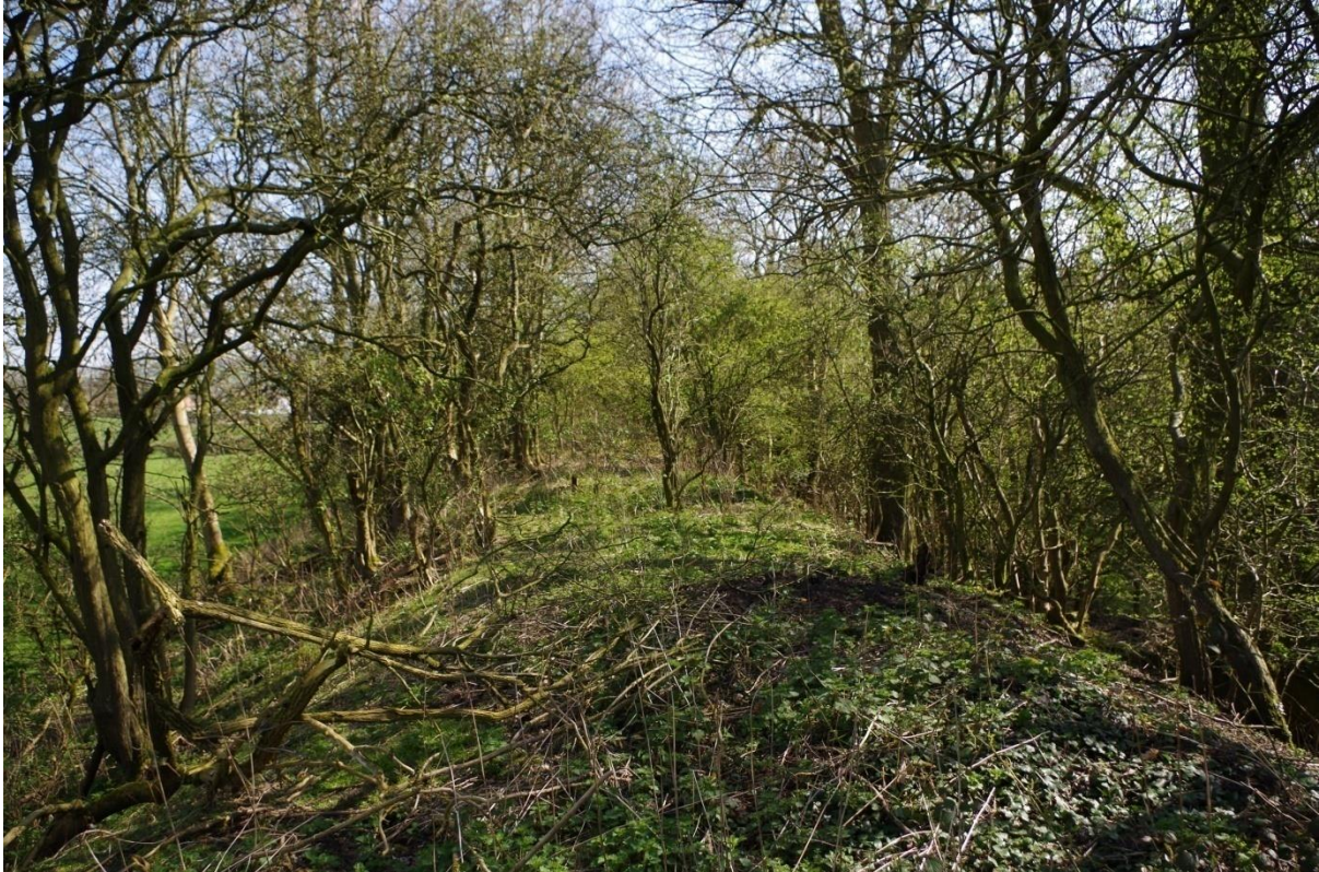
Plate 13. (Above). The overgrown embankment of the south Etherley Incline, looking south towards St Helen Auckland.
