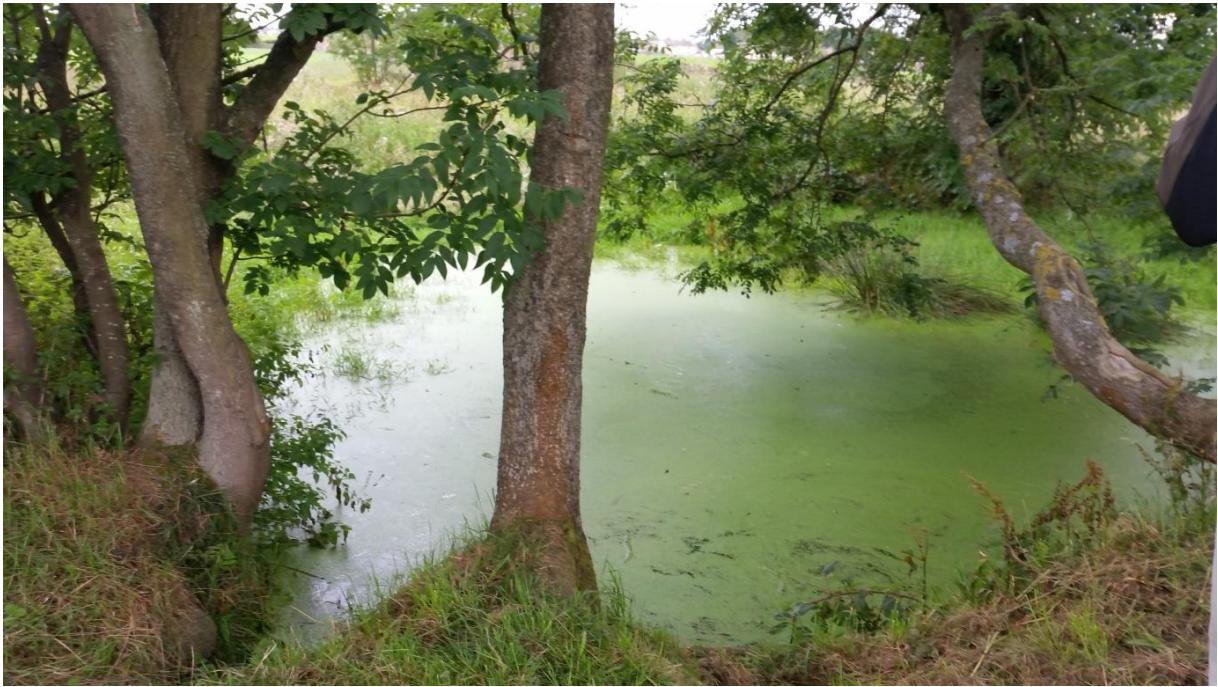
Plate 8. The remains of one of the reservoirs that fed water to the Etherley Engine House
