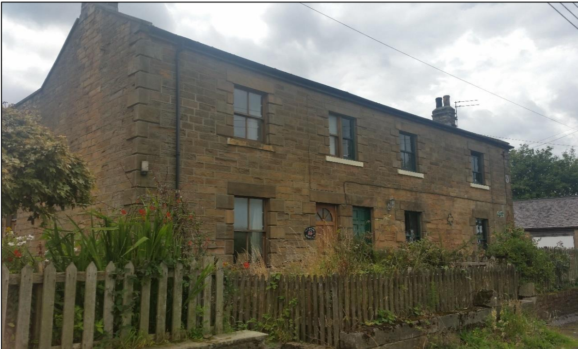
Plate 16. The engineman's house with the blacksmith's house (?) adjacent from the north
