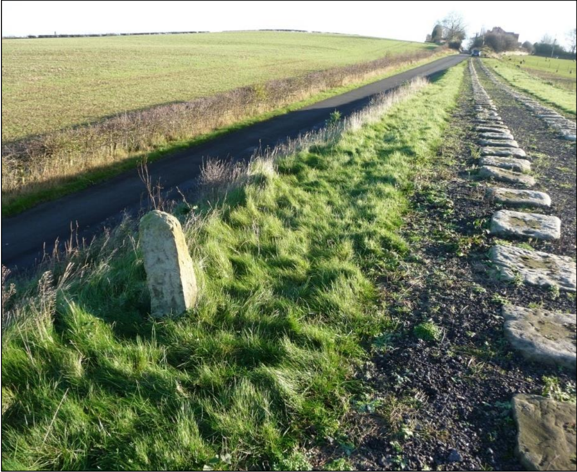
Plate 12. The Brusselton Incline looking east with extant sleepers and an S&DR milestone
