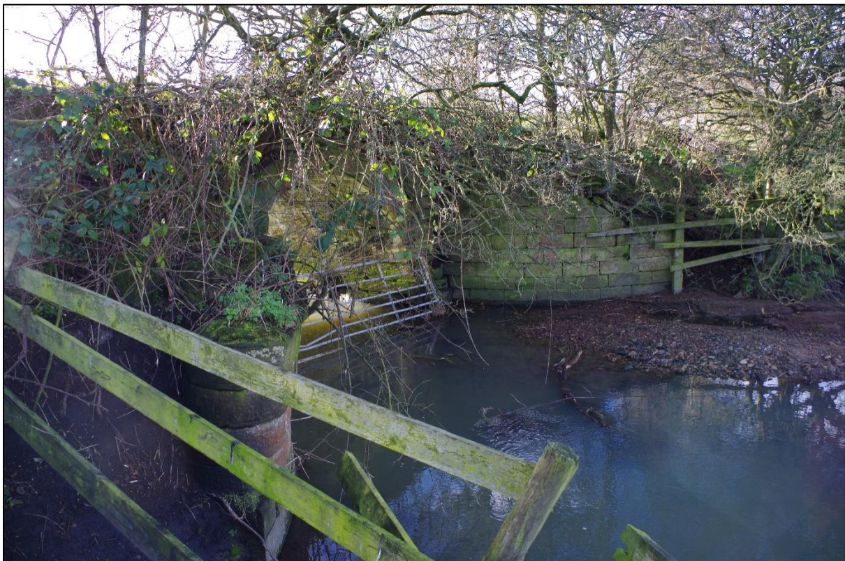
Plate 6. The north side of Hummerbeck Bridge.
