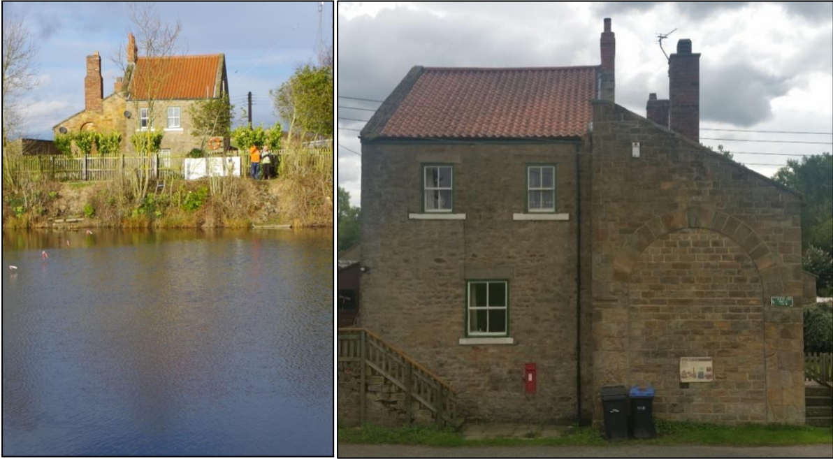
Plate 15. The Engine House seen from the south across the reservoir (above left), and from the north (above right)
