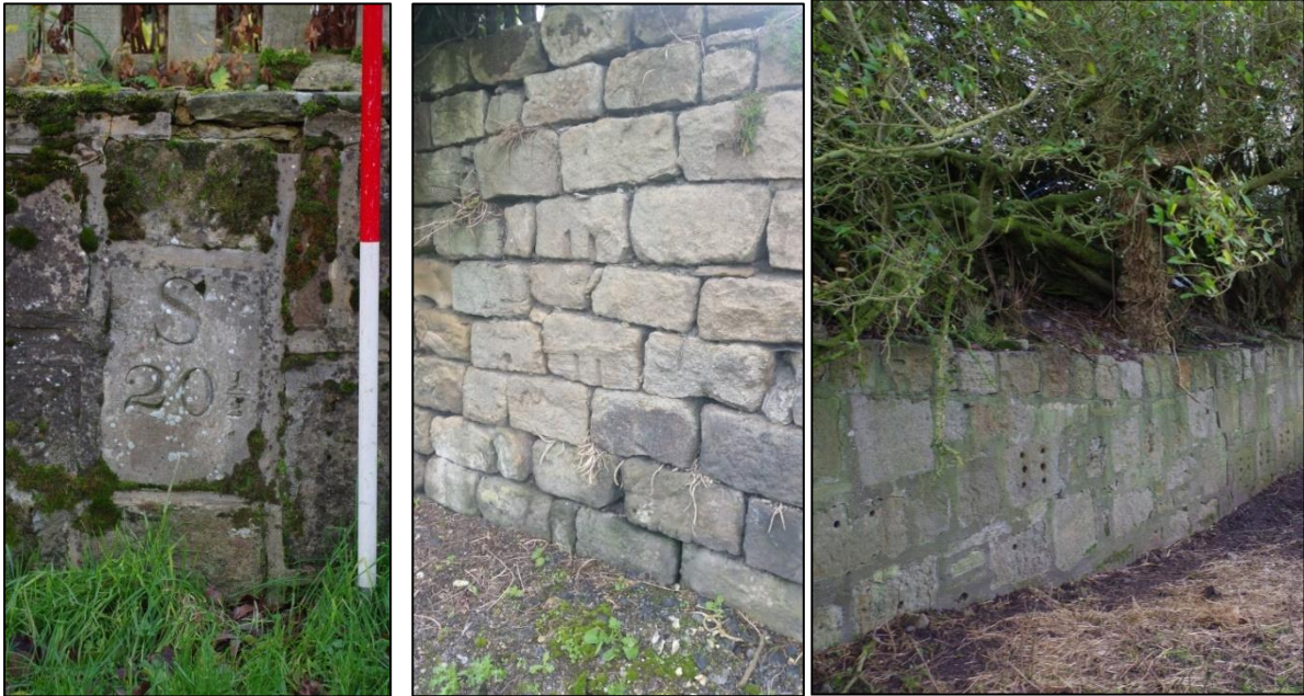
Plate 17. (Left): The S&DR Milestone marking 20 ½ miles to Stockton and now incorporated into a garden wall of the Engineman's House. (Centre): split stone sleepers reused in the garden wall of the Engine House. (Right): the walls of the reservoir which also incorporate split sleeper blocks.
