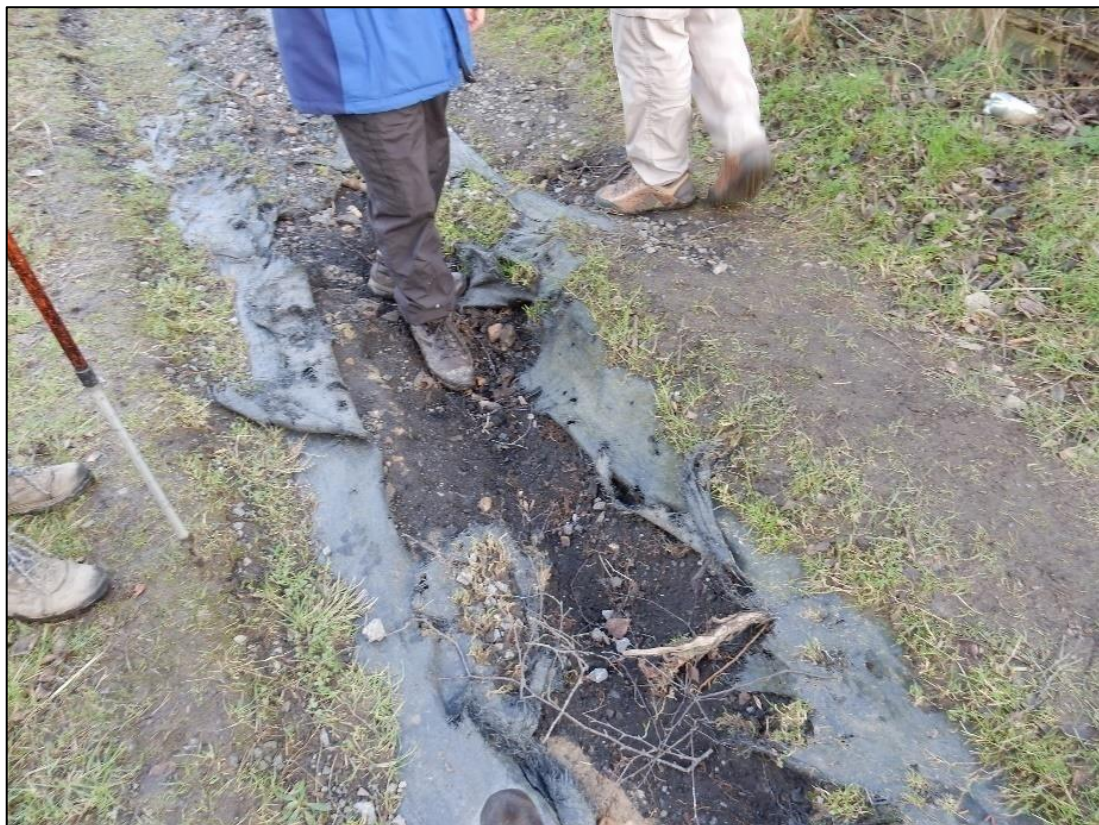
Plate 21. The footpath is worn and needs resurfacing
