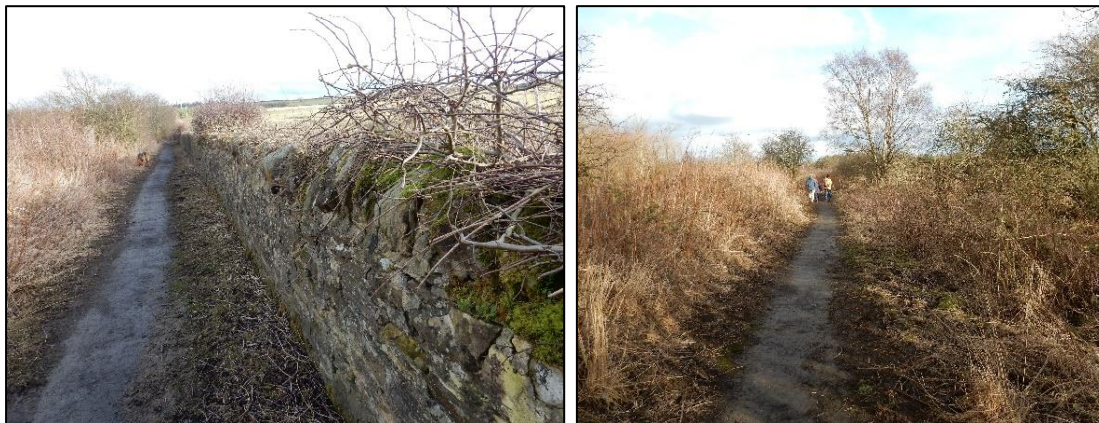
Plate 19. Left: Good quality S&DR boundary walls in places, but the footpath would require widening if more users are to be able to cycle along or use mobility vehicles. Right: Ongoing vegetation clearance will be required to keep the path open
