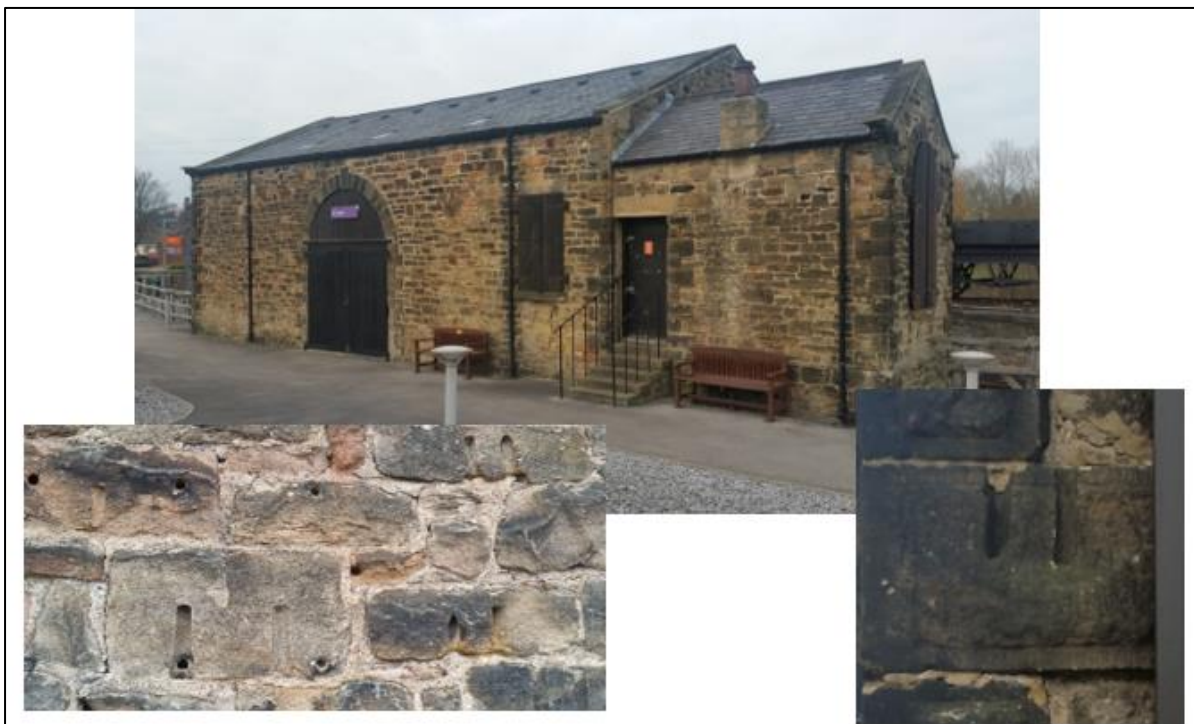
Plate 9. The Goods Shed and detail of reused two hole sleepers in the fabric of the building
