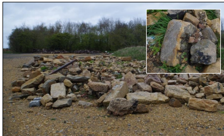
Plate 31. Site of 1825 accommodation bridge recently demolished for Hitachi track improvements (above). Rubble from demolished bridge with re-used 1825 sleeper stones (inset). Line south from Millennium Way, note the small stone retaining wall at base of cutting an original 1825 design feature (above right).
