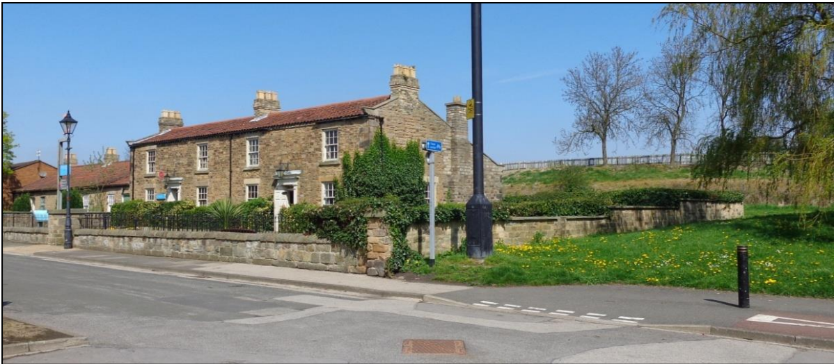
Plate 13. Hackworth's House and adjacent cottages. The green area to the right is the site of the workshops seen in plate 11.
