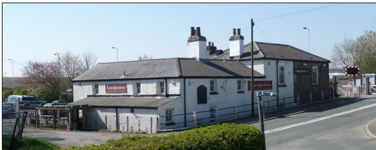
Plate 27. The Locomotion One public house today.
