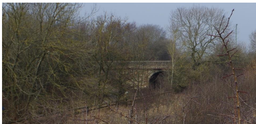
Plate 23. School Aycliffe Lane bridge, the south side of which is built in a style congruent with 1825.
