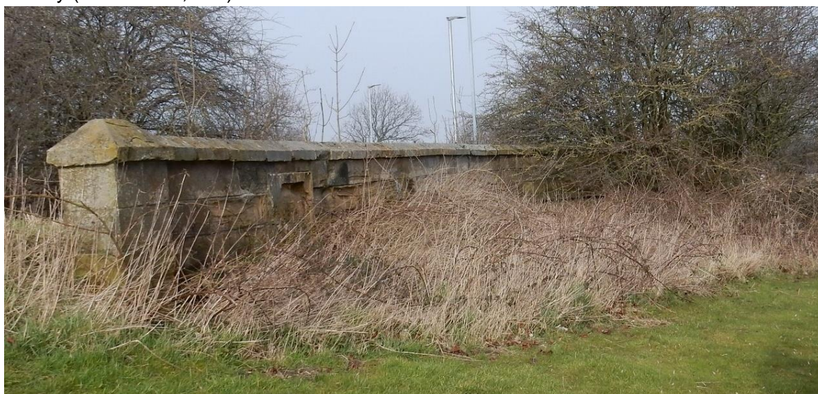
Plate 22. The disused and backfilled bridge serving the Clarence Railway
