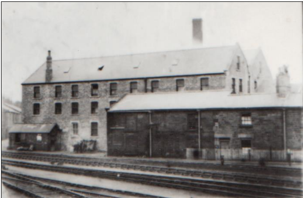
Plate 4. A terrace including Hackworth's first house in New Shildon in the foreground with an engine works building to the rear (photo courtesy of Jane Hackworth-Young)
