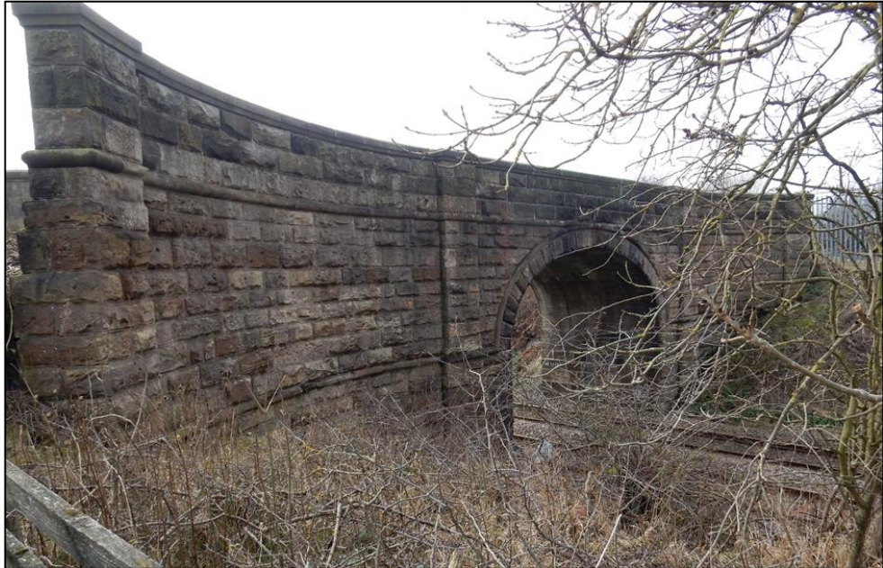
Plate 23 Aycliffe Wood House Bridge.
