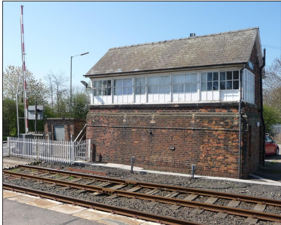
Plate 28. Heighington signal box of 1872. The bricks are noticeably different where it was extended c1912.
