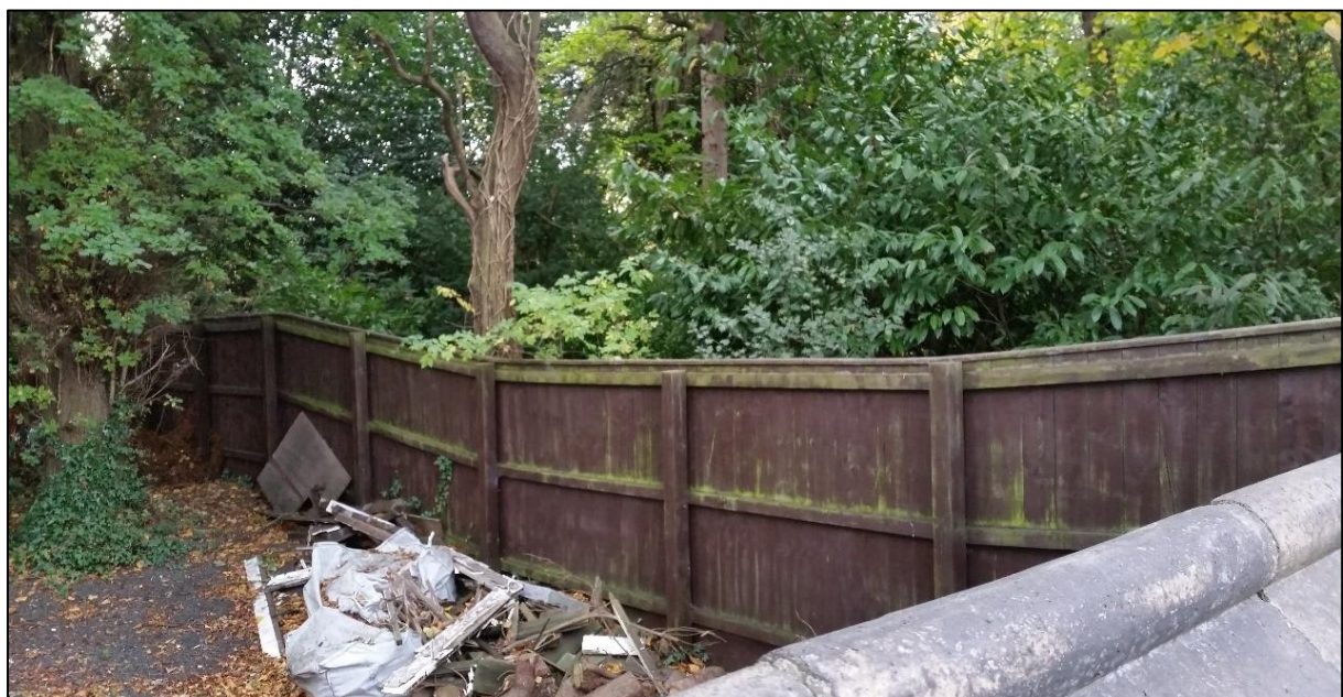
Plate 8. A dip in the fence line of a front garden on Yarm Road marks where the S&DR railway cutting was and so it may still survive buried below ground in the front gardens of many properties along this stretch.
