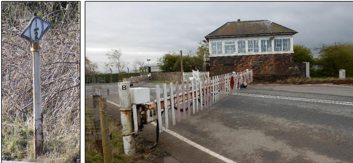
Plate 6. Left: later cast metal distance marker. Right: Urlay Nook signal box from the north.
