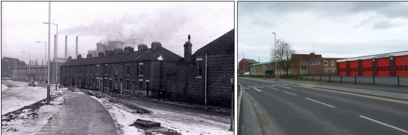
Plate 24. Left: This image dating to 1968 shows the works to create the ring road and the new police station, with existing street frontage housing due to be demolished where the fire station is now (image courtesy of Chris Lloyd of the Northern Echo). Right: Unfortunately, the open spaces and modern buildings which replaced the terraced housing are devoid of character and further emphasise the separation of Parkgate from the town centre
