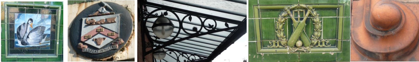
Plate 17. It is the small decorative details that combine to make Parkgate of architectural and artistic interest. The palette is rich in glazed terracotta and green glazed tiles
