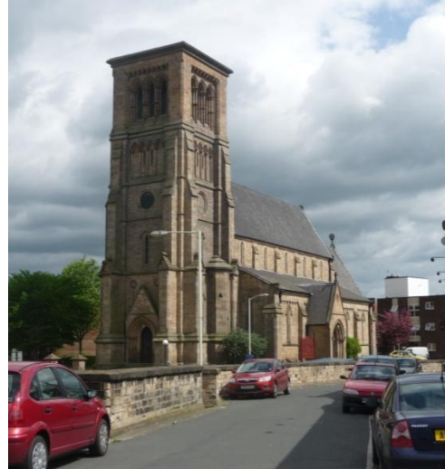
Plate 10. St. John's Church (also known as the Railwayman's Church) by John Middleton as published in 1854 showing the spire that was intended and, left, in 2013 – the spire was never built. The same view is no longer possible due to increased urbanisation.
