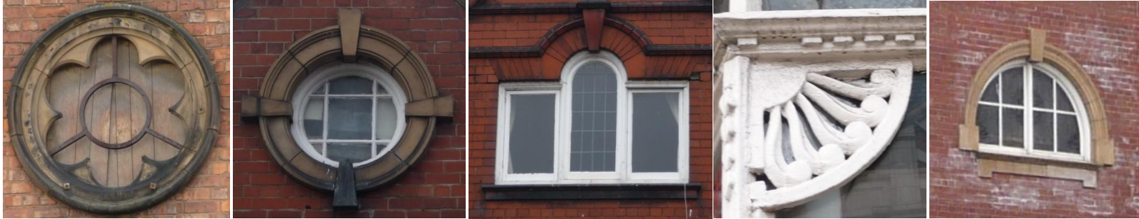
Plate 15. Few traditional windows have survived in this area, but those that do are predominantly 1904-8. Windows are in a variety of shapes, although the circular and lunette are especially popular amongst the red brick Edwardian buildings. Shop front windows have retained their small scale and where they survive, are mostly 1920s-30s; most are in urgent need of conservation.
