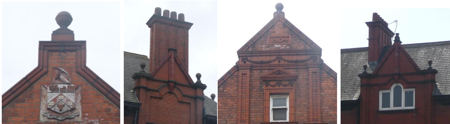
Plate 16. Distinctive gable features in Parkgate using (glazed) red brick and including tall chimneys, using window detailing, string courses, ball finials, swags, crests and pilasters to add interest
