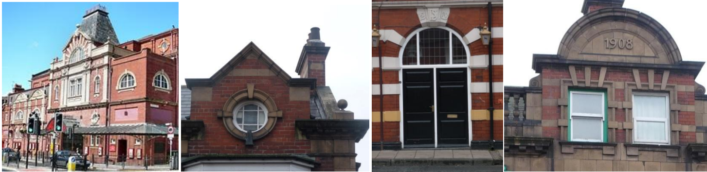
Plate 12. The details from the Civic Theatre are to be found in other properties on Parkgate. Most buildings are of brick with sandstone detailing, but many also make use of glazed brickwork, interesting gable features, circular and semi circular windows , starburst and starburst derivatives and art nouveau date stones.
