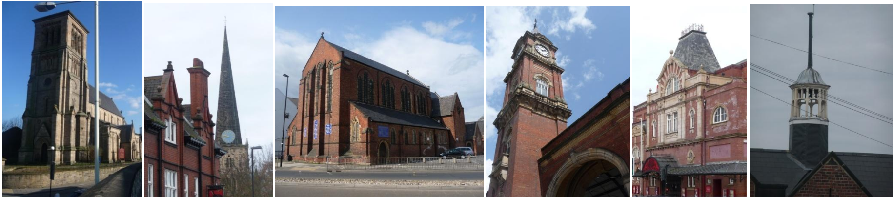
Plate 6. Landmark buildings in or near the conservation area which provide prominent architectural features and roofscapes worthy of conservation. (Left to right: St John's; St. Cuthbert's (outside the conservation area); St Hilda's, Bank Top Station (outside the conservation area) and the Civic Theatre
