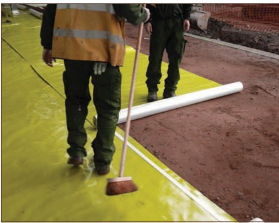
Figure A4.15 LDPE type gas membrane overlap and double sided tape. Sand blinding to protect underside of gas membrane (courtesy A Proctor Group)
