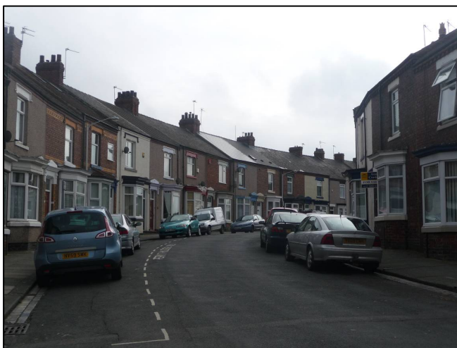
Plate 17. Montrose Terrace gently curves to form a crescent but it has lost its original harmony created by matching brick facades with the same brick detailing and the same window and door styles now hidden behind render and pebble-dash (colours would always have varied).
