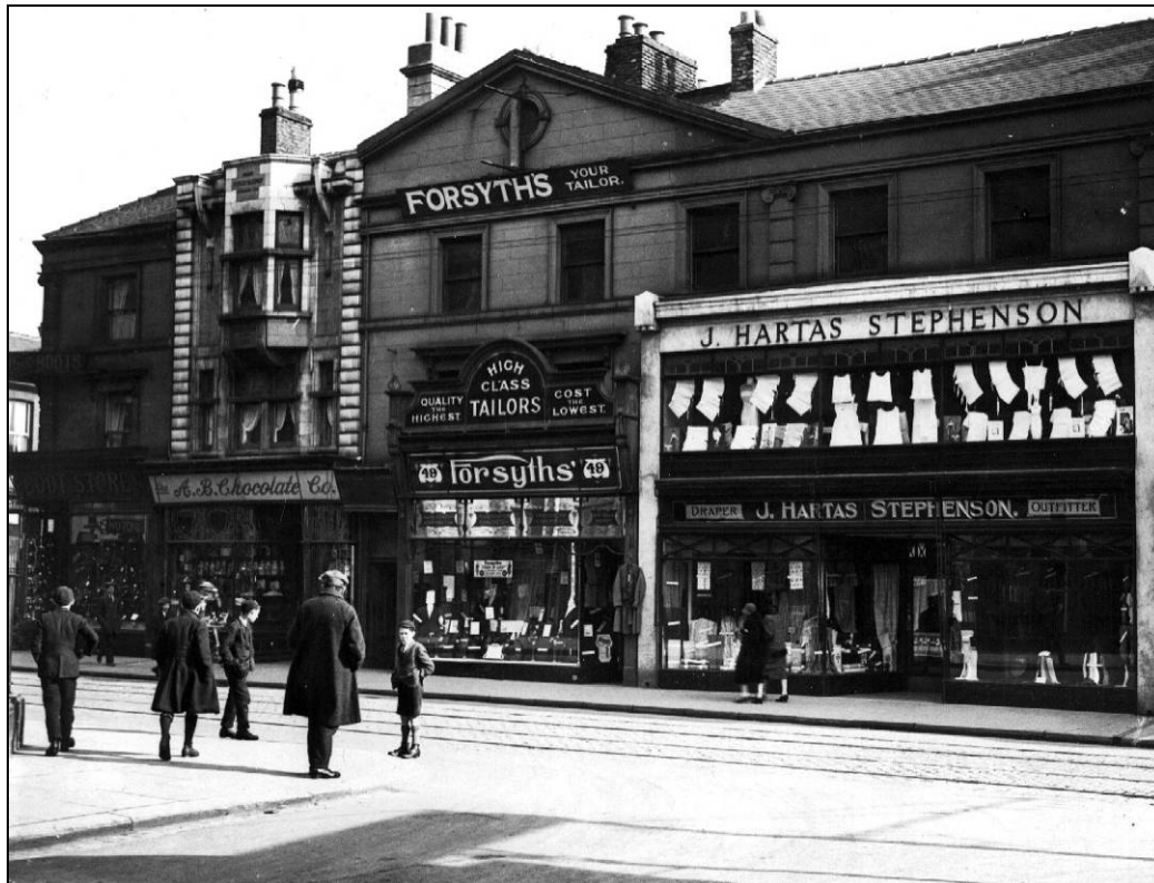
Plate 1. Edward Pease's home on Northgate. By the 1930s the grand classical façade had been divided up at ground level with shop fronts and a tiled façade added to one bay in 1907.
