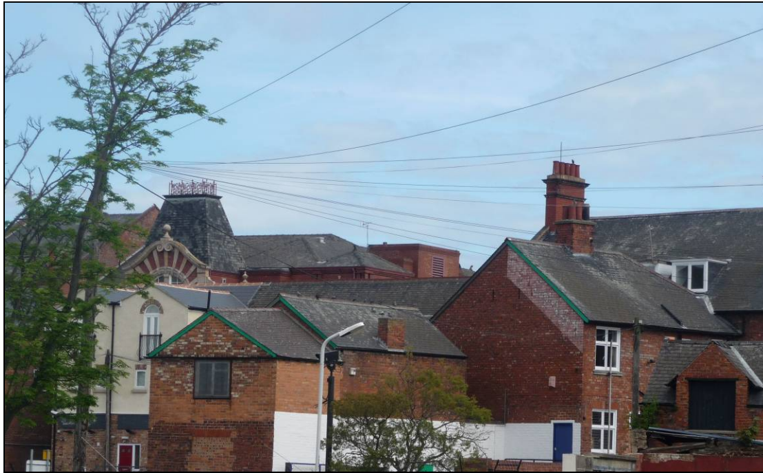
Plate 13. The back views of terraces provide an eclectic mix of roof lines and extensions which display the archaeology of development
