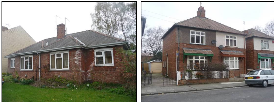
Plate 21. Bungalows for the 'aged' were built by the council in 1937 on St Hilda's Street and were part of a move away from terraced housing towards larger plots with gardens, based around a cul-de-sac. The 1930s saw semi detached houses springing up throughout the suburbs but here on Lodge Road they were used as infill amongst existing terraced development. These houses were built by Dunwell who bought a tract of land between here and East Mount for development (C. Fish pers comm.)
