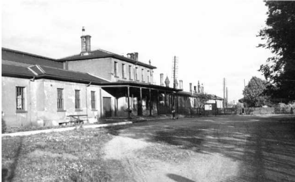
Plate 32. North Road station in 1936
