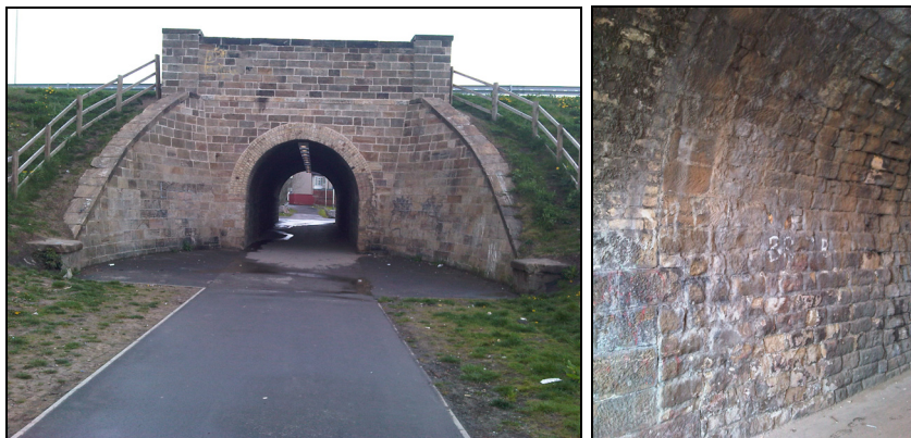
Plate 47. The cow tunnel today is encapsulated in a modern tunnel (left) but the join where it becomes the original S&DR cow tunnel can still be seen inside (right)
