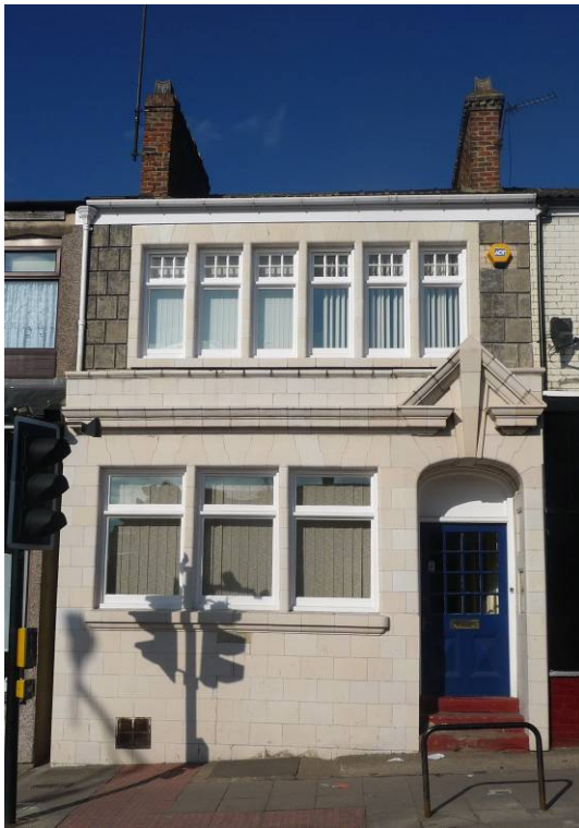
Plate 31. The labour party offices on Victoria Road in 1983, now the home of Groundwork
