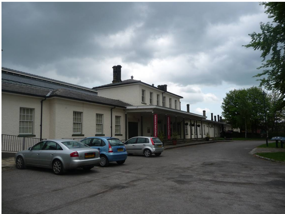
Plate 33. North Road station (Head of Steam Museum) in 2010; its role as a museum and its listed status is clearly benefitting the conservation of the building
