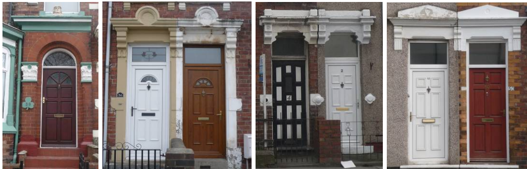
Plate 16. Ostentatious doorways: East Mount Road (left and second left), Haughton Road (centre right) and Montrose Terrace (right). These doorways all display the appearance of having off-the-peg decorative additions designed to attract 'better class' customers by a speculative builder. Sadly few of the doors themselves are original designs and now detract from the fine surrounds
