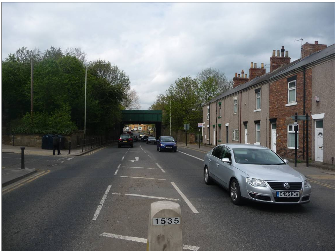
Plate 45. The viaduct in 2010
