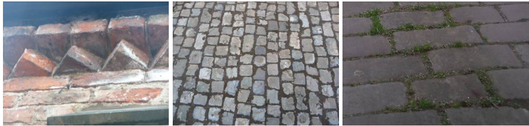
Plate 27. Distinctive building materials in the town centre fringe: red brick for boundary walls and buildings, often with detailing, scoria blocks for back lanes and drains, and stone blocks for back lanes – all locally sourced
