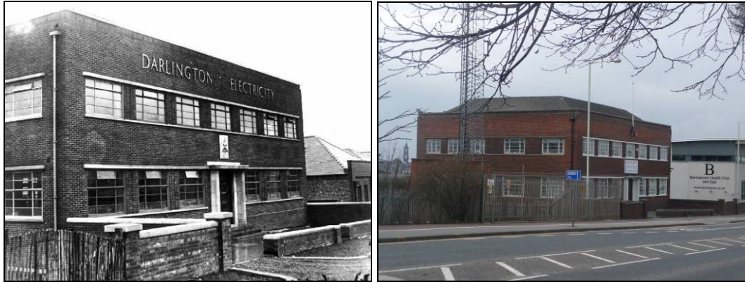
Plate 23. A 1930s building (Darlington Electricity in the 1930s) on Haughton Road with its typical low wide windows with horizontal metal glazing bars which contrast with earlier Edwardian and Victorian styles of tall narrow windows in timber. It retains the use of brick with stone detailing however. The old coat of arms pictured in the black and white photo remains boxed-in behind the modern sign and is a splendid piece of coloured tile or faience (I. Dougill pers comm. (12.7.10))
