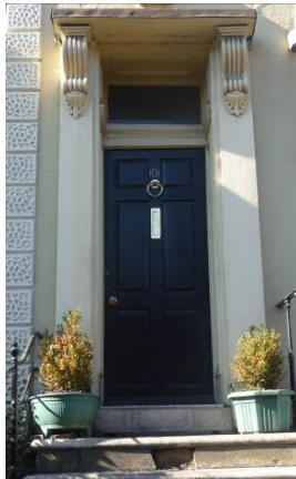
Plate 15. 101 High Northgate with a six panel door and classical style which reflects earlier Georgian fashions
