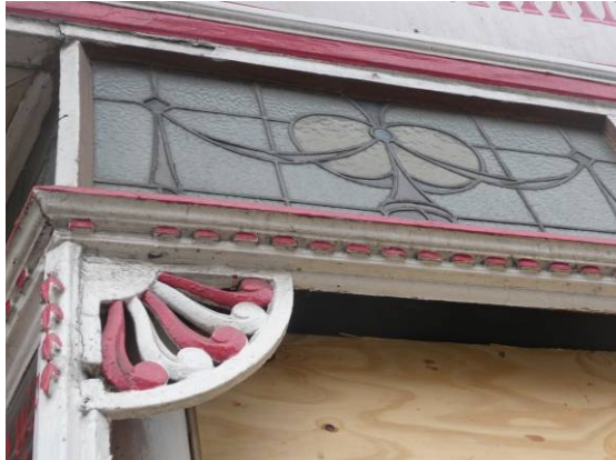
Plate 10. Early 20 th century shop front detail on Parkgate
