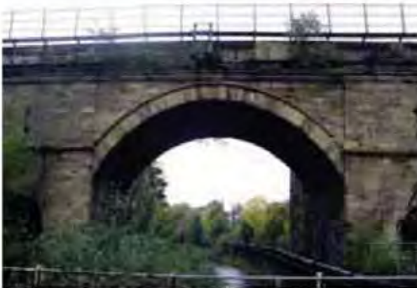
3. Skerne Bridge, a scheduled Ancient Monument. (SAM)
