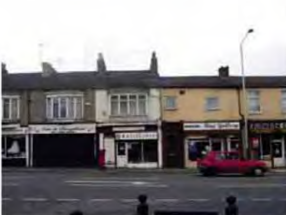
29. Original window and door openings have been replaced, and a poor state of repair prevails (High Northgate).
