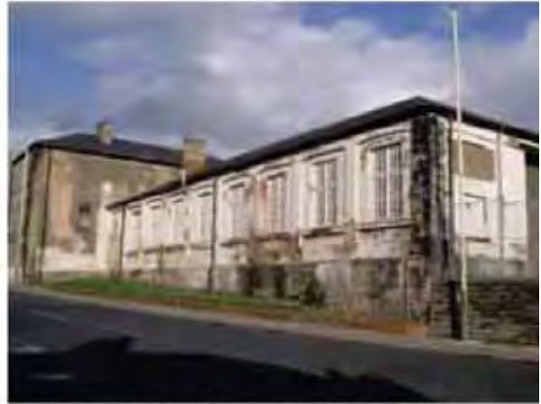
2. The former S&DR Carriageworks (Grade II) strongly defines the boundary of the area. Now occupied by the A1 Steam Locomotive Trust.
