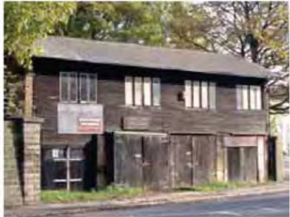
16. The former lime cells at the junction of Hopetown Lane and Station Road, (Grade II)
