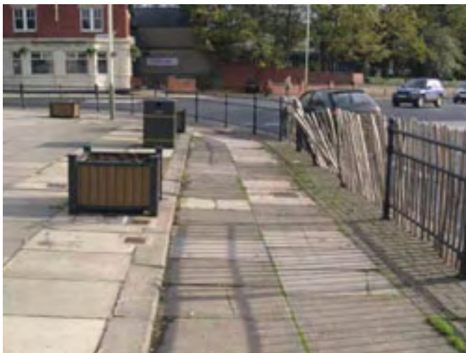
15. Elements of street furniture are in poor state of repair.
