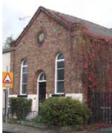
6. 92 the Green; a former Chapel which is a positive feature in the street scene.
