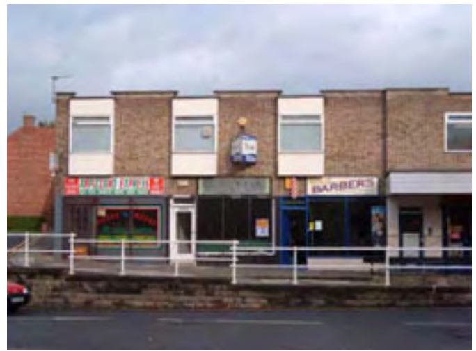
16. The modern shop frontages of 28-36 are located directly opposite the listed 19, 39 and 39a Cockerton Green
