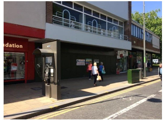
Photograph 10: Former McDonalds unit, Northgate
