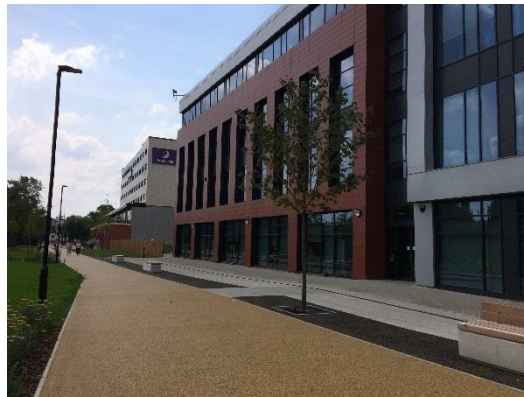
Photograph 5: Ground Floor, Feethams
