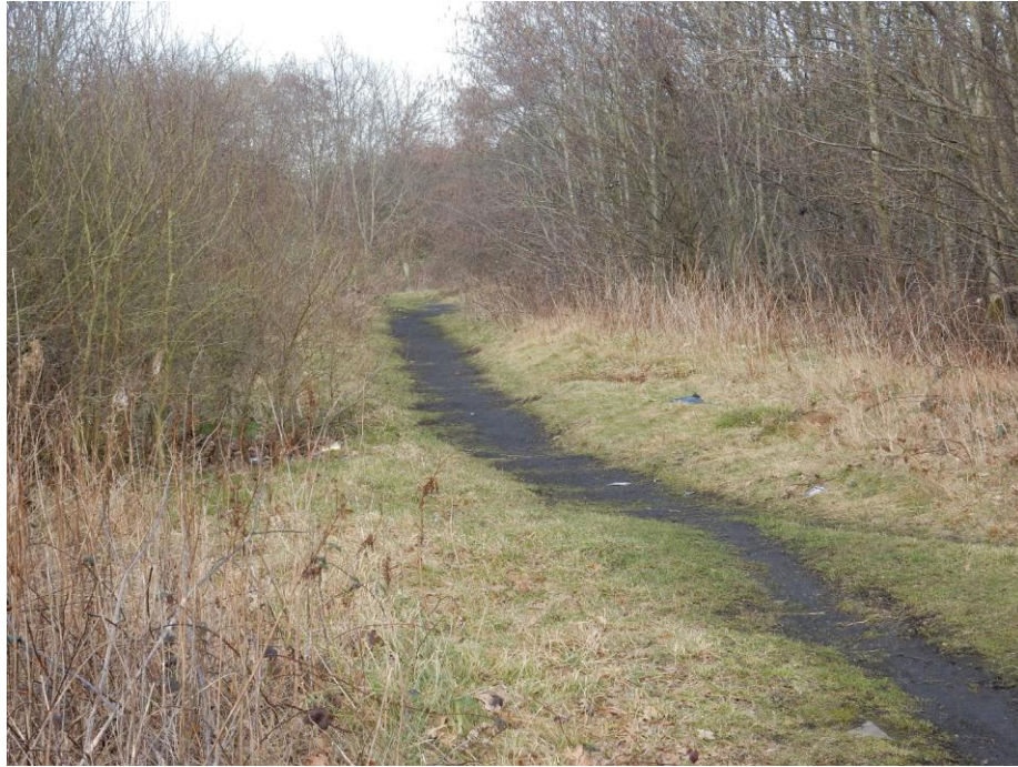
Figure 43. The route of the Croft branch line. Differential drying conditions highlight the ghosts of wooden railway sleepers running across the track
