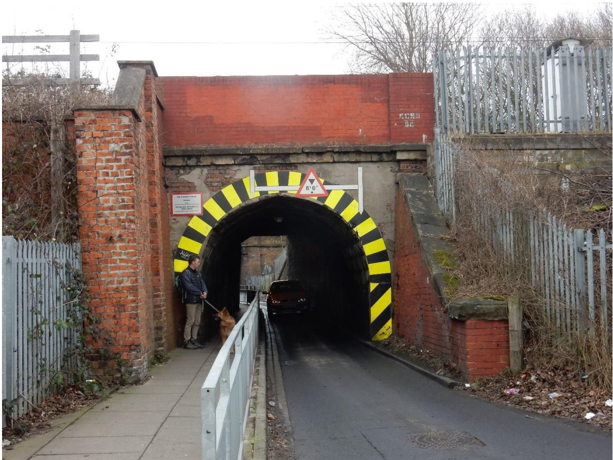
Figure 36. Parkside Bridge west side 2019
