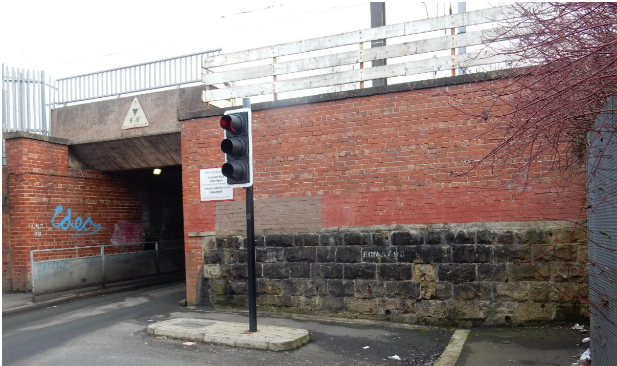
Figure 33. The bridge on Smithfield Road. A modern replacement but incorporating earlier stone walls which have reused sleeper stones from 1829 used as building materials
