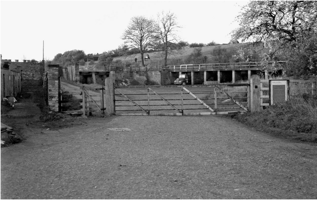
Figure 71. The Coal Drops and Yard Gates at Croft Depot in 1964 just before closing (photo R. V. Webster)
