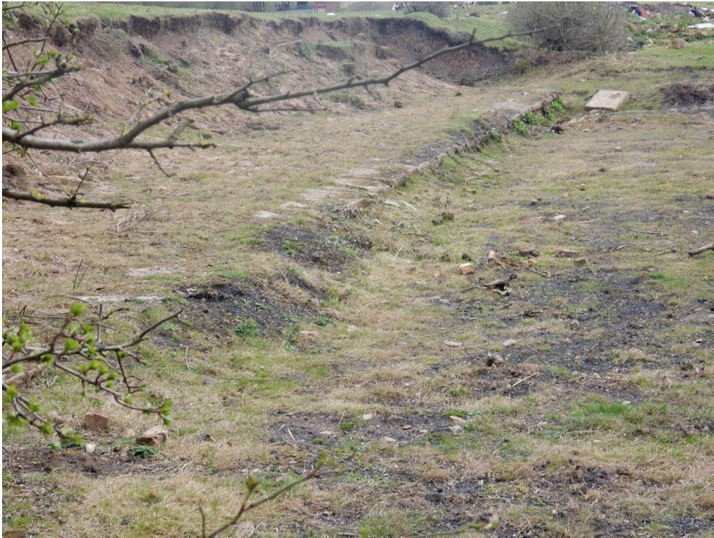
Figure 53. Detail of the stone revetments along the trackbed
