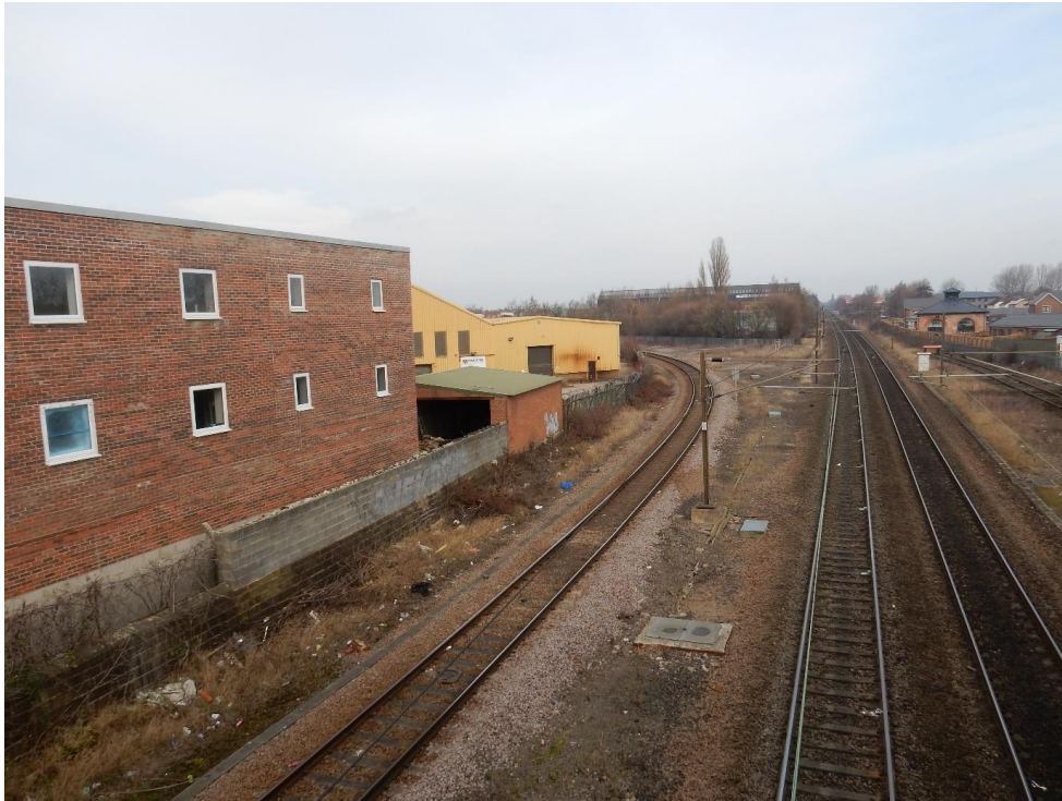
Figure 16. View north towards the curve on the Croft branch line from Houghton Bridge. The GNER Engine Shed can be seen top right. The tracks on the right are the East Coast mainline. Just beyond the Engine Shed, the mainline of the S&DR runs east-west across the mainline and has been commemorated with a metal sign since 1925. The buildings to the left are on the site of the late 19 th century Houghton Bridge Wagon Works.
