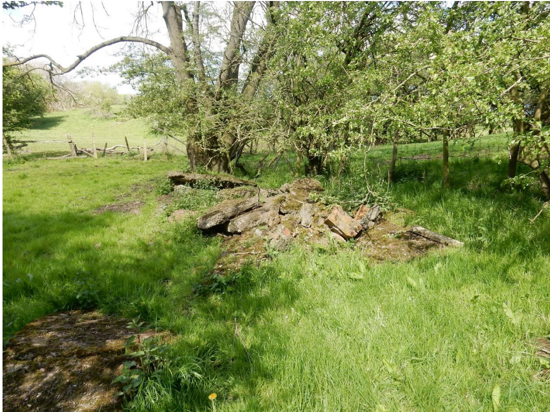
Figure 64. Demolition debris near Black Banks
