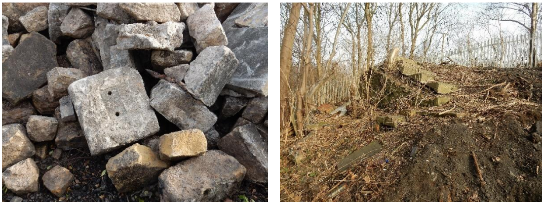
Figure 11. Left: two-hole sleeper blocks presumably originally from the 1829 trackbed and now part of demolition debris at John Street (S&DR 827). Right: the fragmentary and broken remains of buildings at the west end of the sidings north of John Street and due to be developed (S&DR 833).
