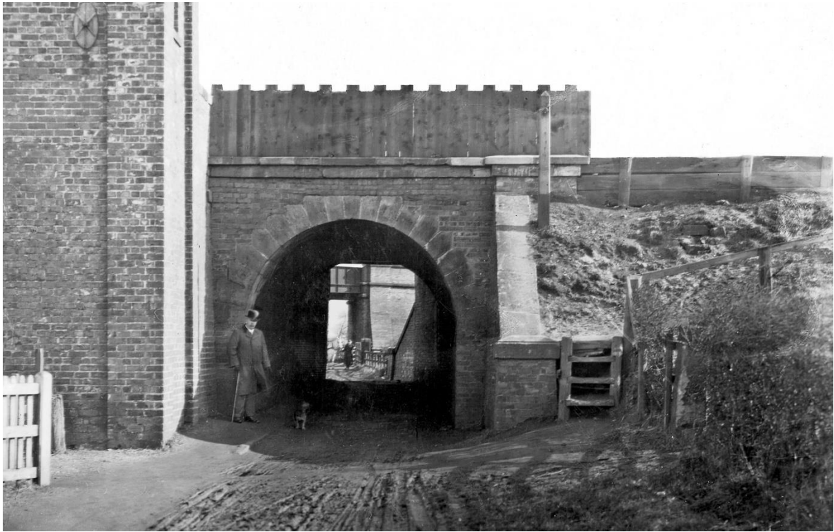
Figure 35. Parkside bridge west side (Centre for Local Studies, Darlington Library)
