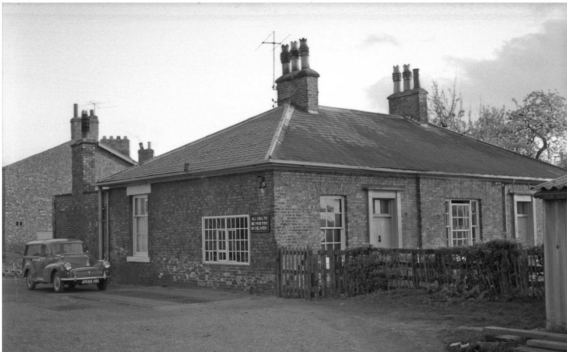
Figure 70. The weigh house and probable accommodation for the depot agent (no evidence of this building surviving, it appears to have been demolished to build Linden Court's predecessor buildings). To the rear was the weighbridge also now demolished (photo: R. V. Webster)
